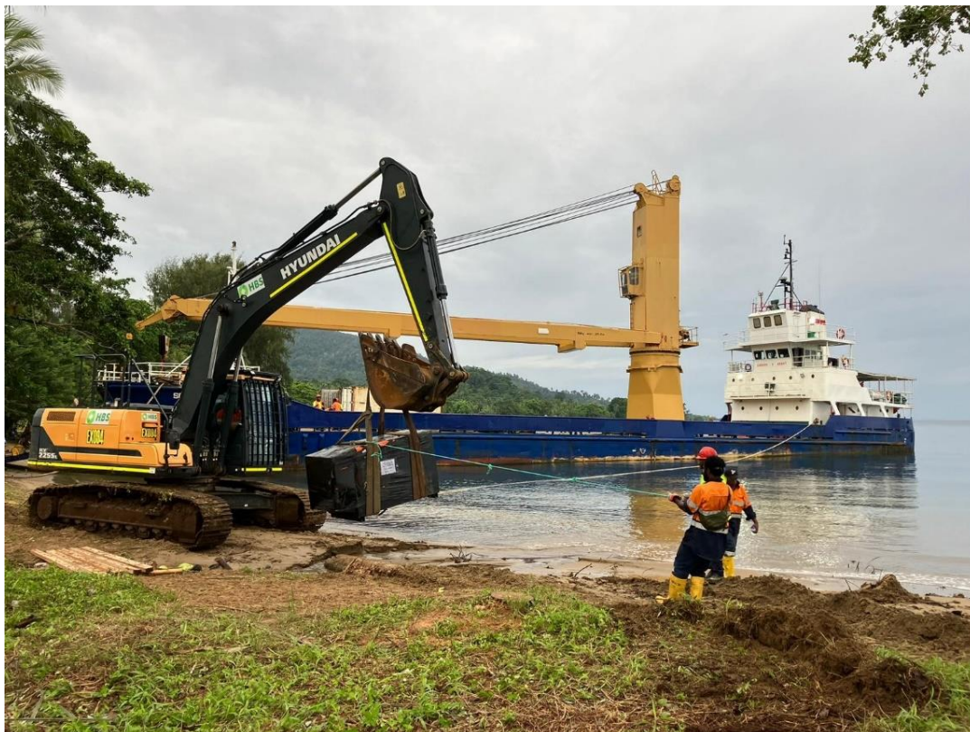
Figure 6 Barge 'Sea Swallow' - mobilisation of earthmoving equipment and supplies, March 2024
