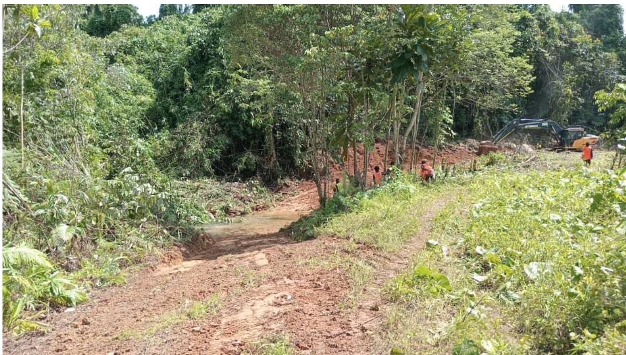
Figure 7 Track construction, Willie Creek, April 2024
