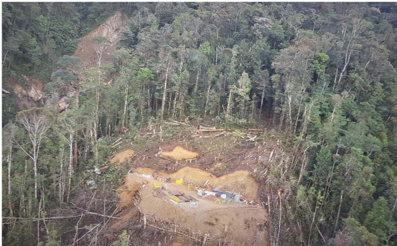
Figure 1 EK002 drill pad in foreground, with Yangkis gold workings in the background – April 2019
